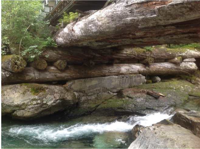
Right Bank Abutment when facing downstream - old crib retaining fill
