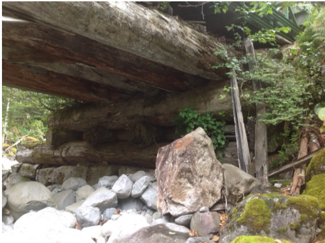
Left Bank Abutment when facing downstream - old crib retaining fill
